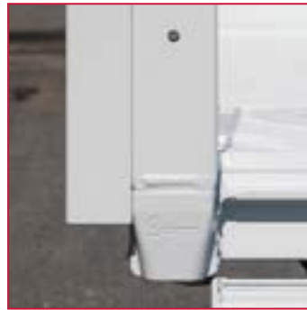
Conical pillar with clamping screw
